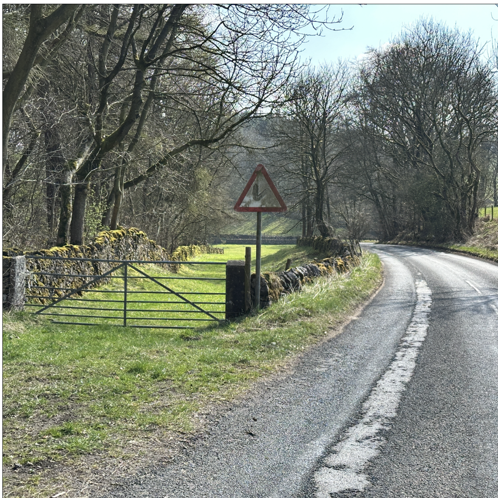
The Turnpike entering Friden Bends at the start of the 1830s embankment which lifts the road over the damp fields of Longdale. The original route ran through the gate to the left.
